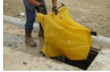
Slide Siltsack® over opposite side of grate.
