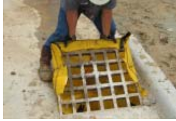
Slide Siltsack® over one side of grate.
