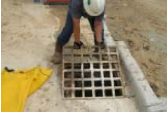
Remove grate from catch basin.
